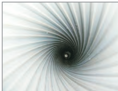
Barrel cleaned after using Vapro 816
